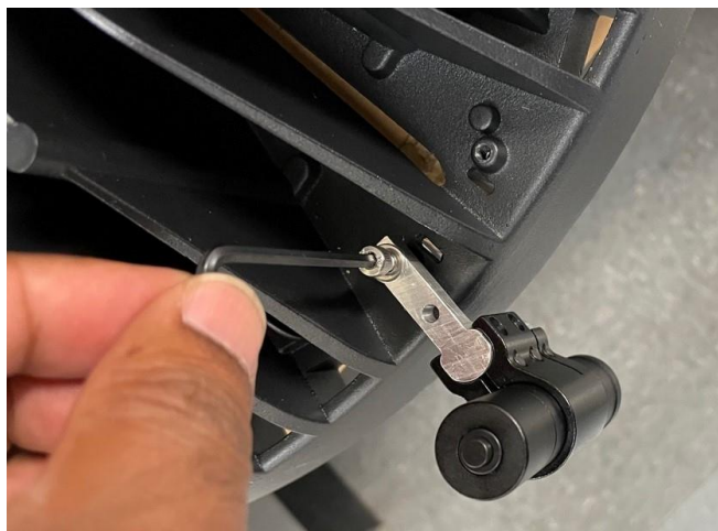
Step 7: Mount the aiming bracket to the fixture using one of the two available screws as shown in the image.
