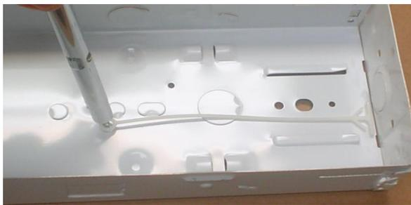
DIAGRAM 1 - Geartray tether placement (in existing fixture)
