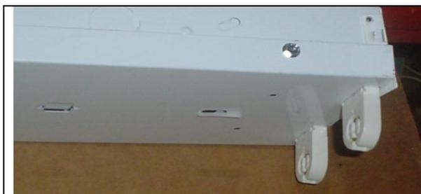
DIAGRAM 5 – Drive tek screw through each of the (4) holes in side of the geartray and into the fixture body
