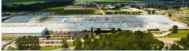
Laurel Transformer Facility
